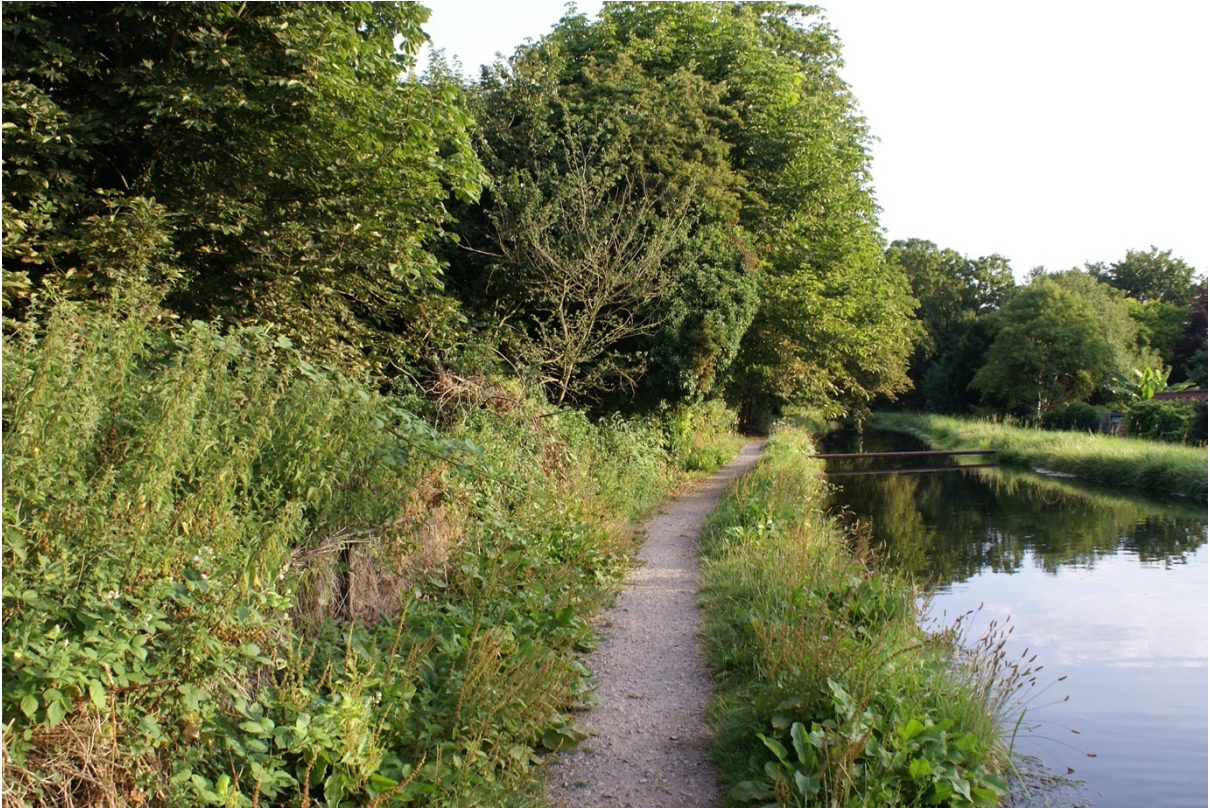
FIGURE 46 LGS3 ST MARGARETSBURY ESTATE BY THE NEW RIVER PATH
