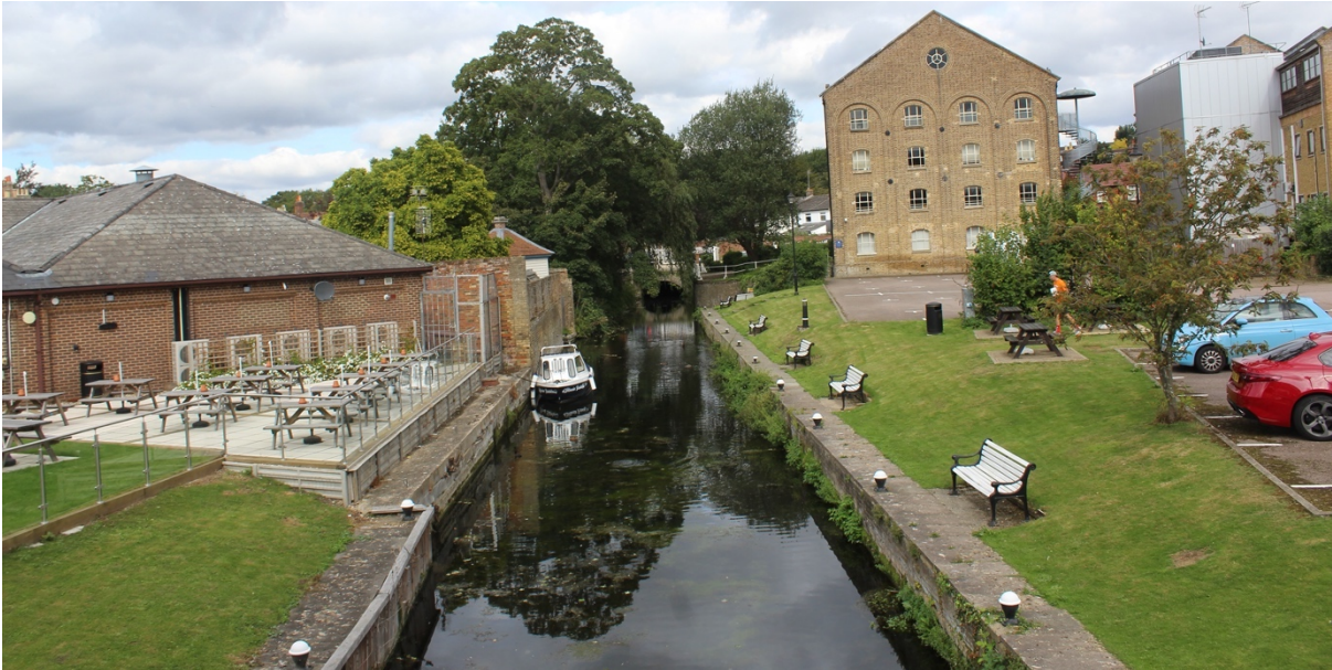
FIGURE 36 VIEW 5 SOUTH ALONG THE MILL STREAM FROM FOOTBRIDGE
