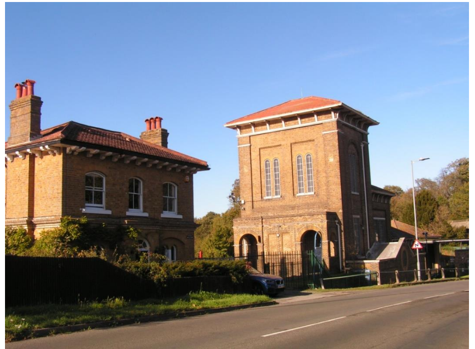
Rye Common Pumping House
